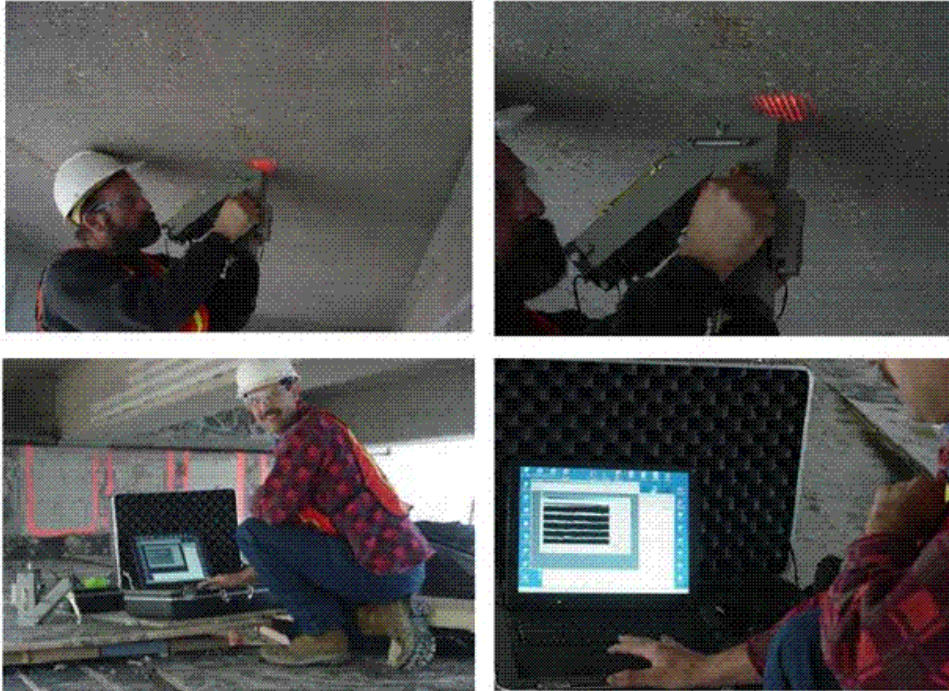
Roughness measurements on the bridge deck
