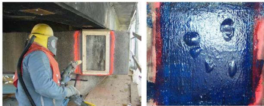
Surface preparation by sandblasting.
